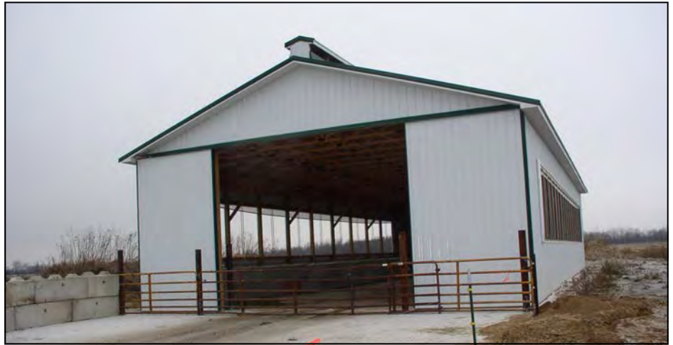
Dry Stack Manure Storage installed by Nathan Allen.
