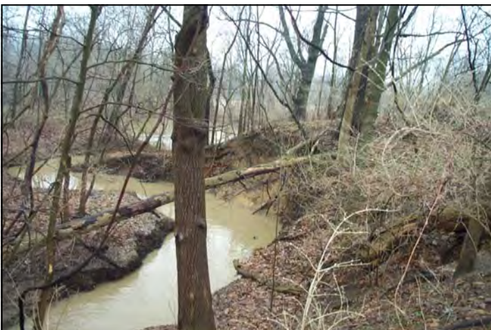
Photo taken of the Townson Drain before rehabilitation in 2008 by the Shiawassee Conservation District.
