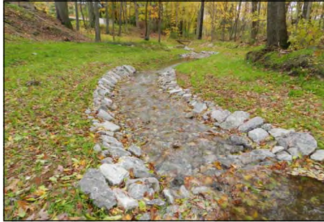
Photo taken after rehabilitation in 2013 by the Shiawassee Conservation District.
